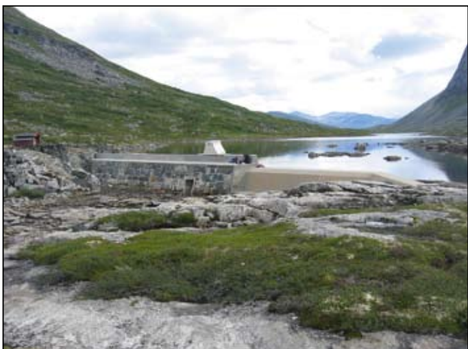
Dam Langvatn, kontroll 2006 08 30
